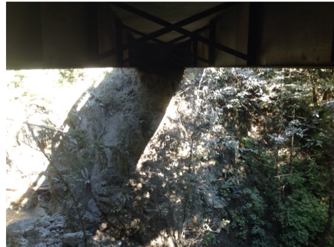
Left Bank Abutment when facing downstream
