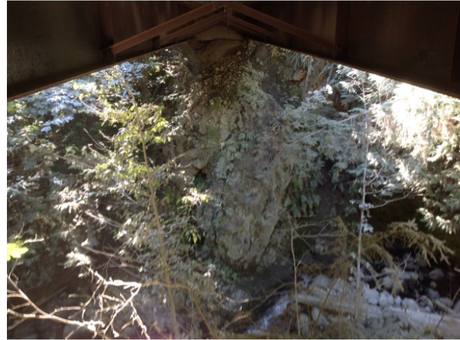
Right Bank Abutment when facing downstream
